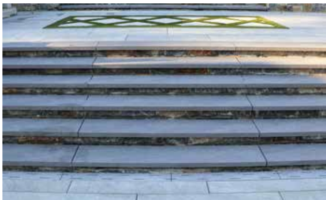
Mitered steps and custom drains
